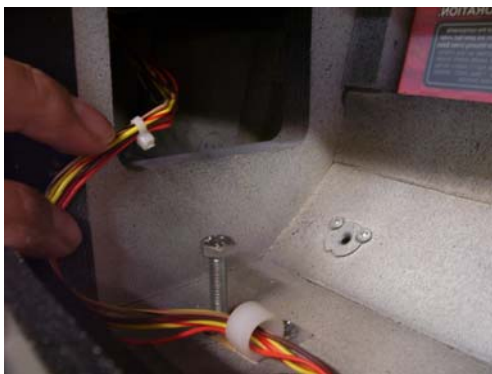
Inside Top Box: Left Side
